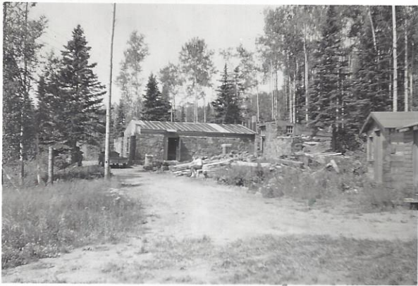
TRINITY LUTHERAN CHURCH at Hovland, Minnesota under construction.
